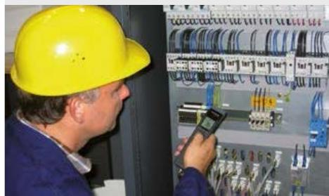
Infrared thermometers are proven time saving tools for predictive maintenance of electrical systems. Check out temperature problems safely with connectors, fuses, electric motors, motor windings, insulations, electrical wiring and electrical cabinets before damages occur.
