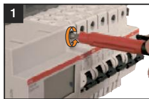
Unscrew the terminal of the installation device
