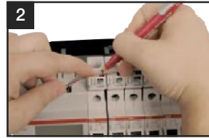
2 Mark the desired placement of the connectors with a pen
