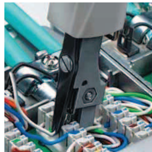
Putting down and cutting the cable in one operation
