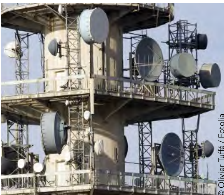
Telecom - Data infrastructure
