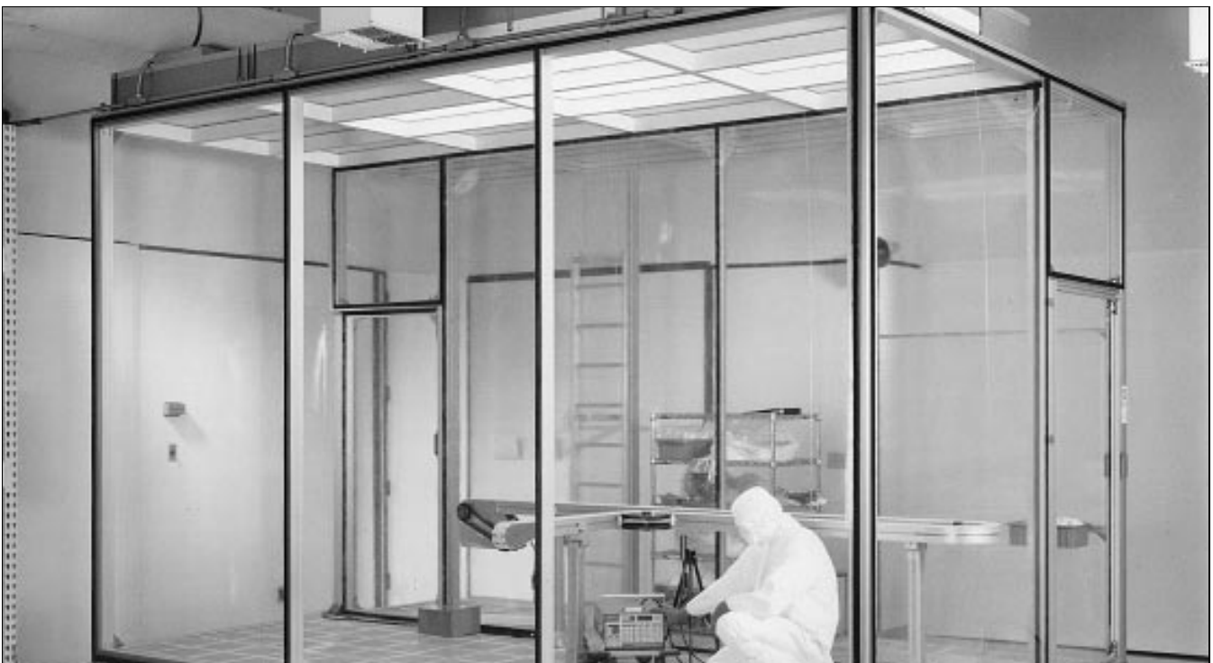
FlexLink structural system XC Clean room for testing of material handling equipment with Class 1 capability.
